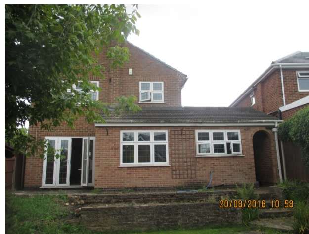
View of north west (rear) elevation
